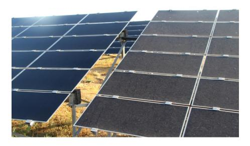
Regular cleaning results in significant efficiency gains
